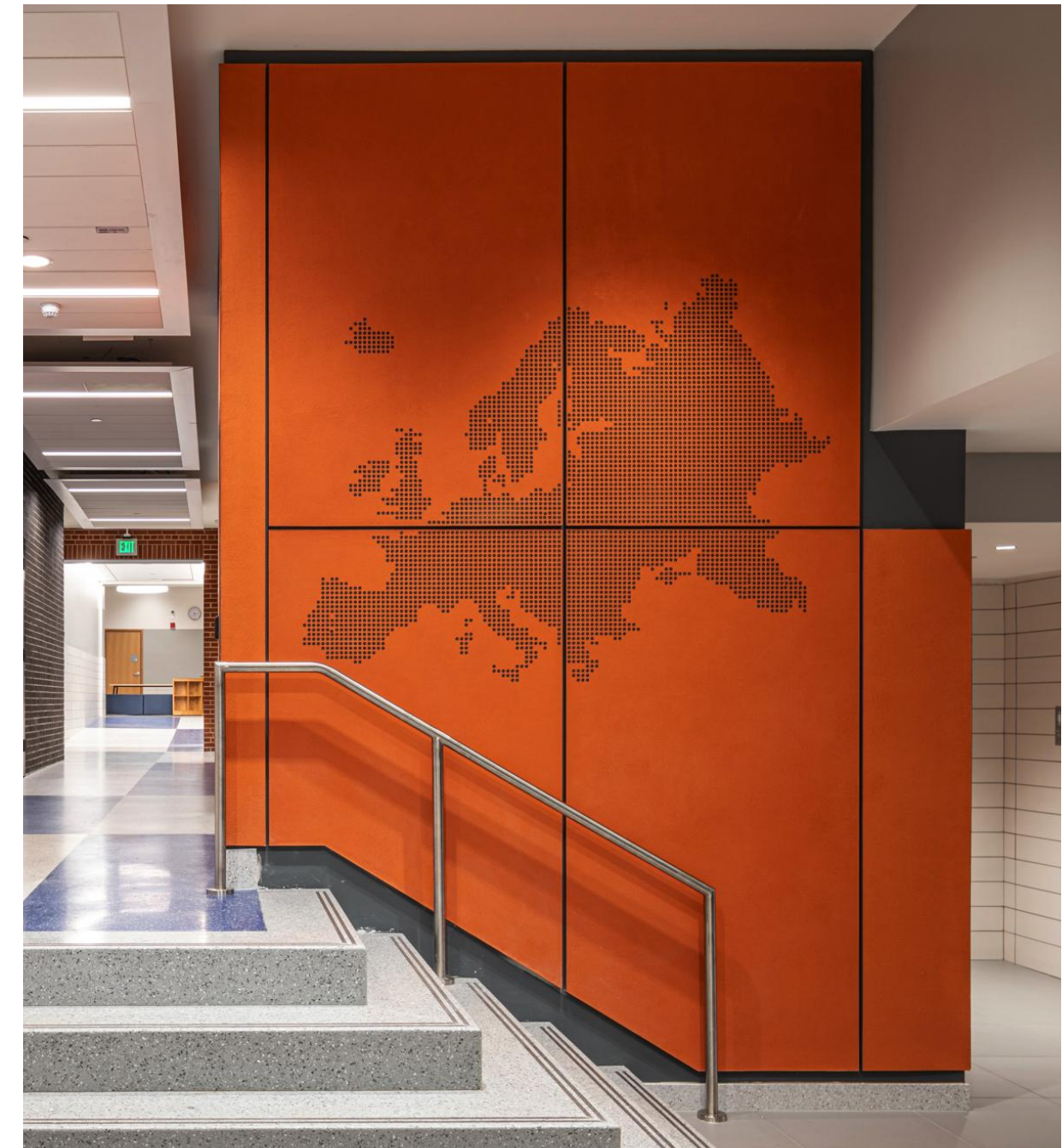
Decorative Plaster Example Installation Eaton Elementary School
